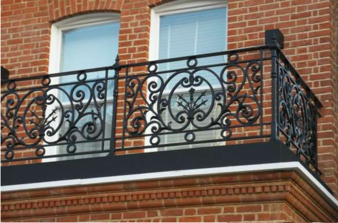
Replica balcony balustrade manufactured and installed by Peter Weldon Iron Designs.
