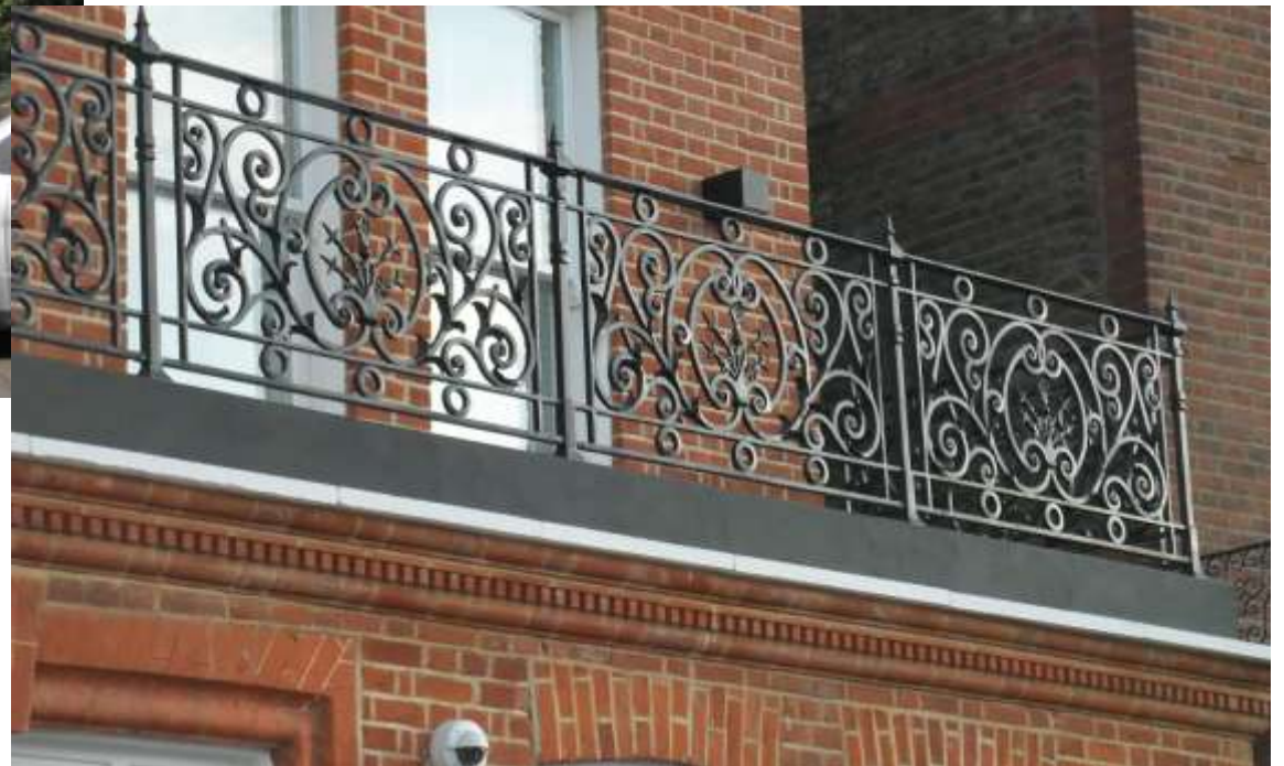
Ironwork by PWID installed.
