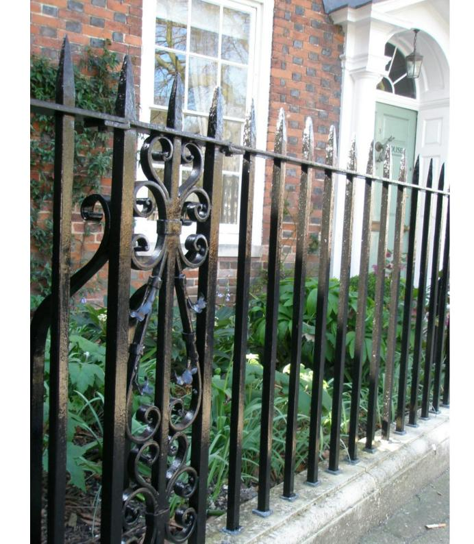
Lead plinths at the base of each vertical section formed by hot lead.
