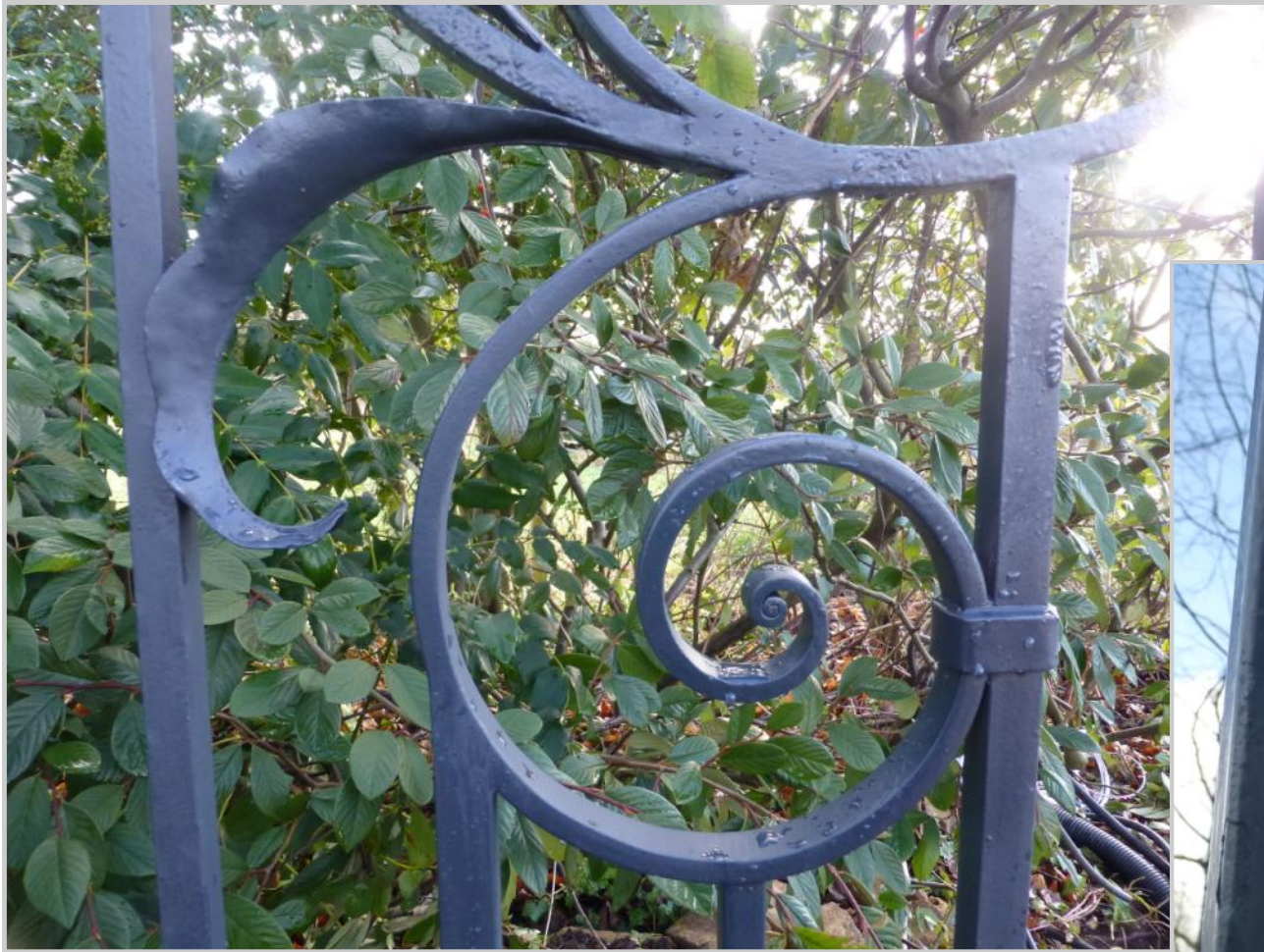
Hand forged scrolls, collars and leaves.
