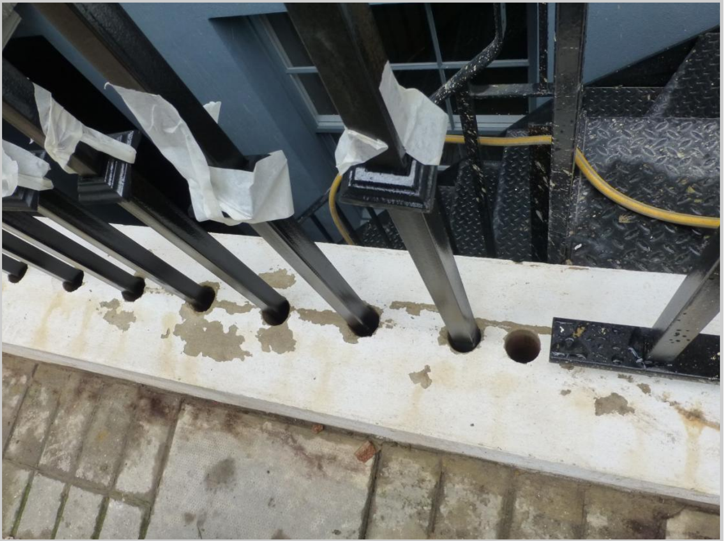
Core drilling into the coping stone in the traditional blacksmith manner.
