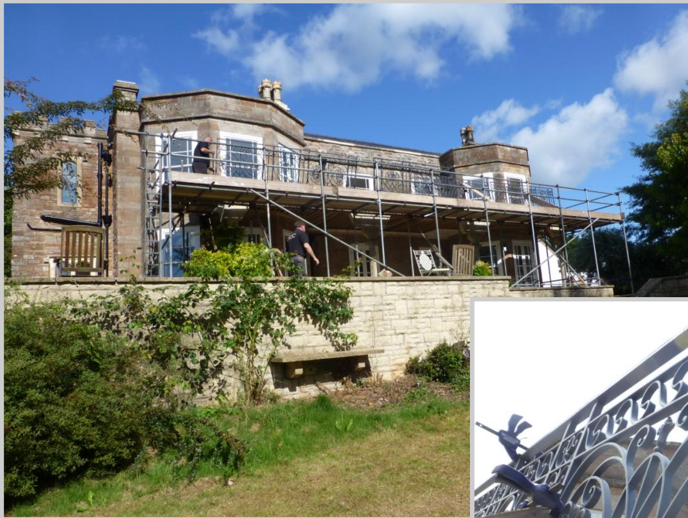
Balustrade during installation.
