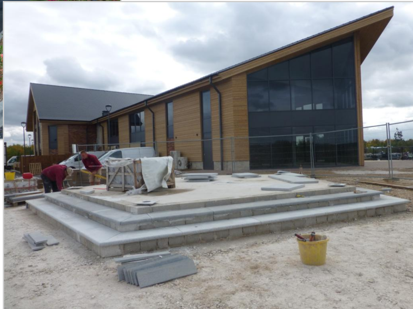
The foundation pad for the event stand is put down by the client prior to delivery.
